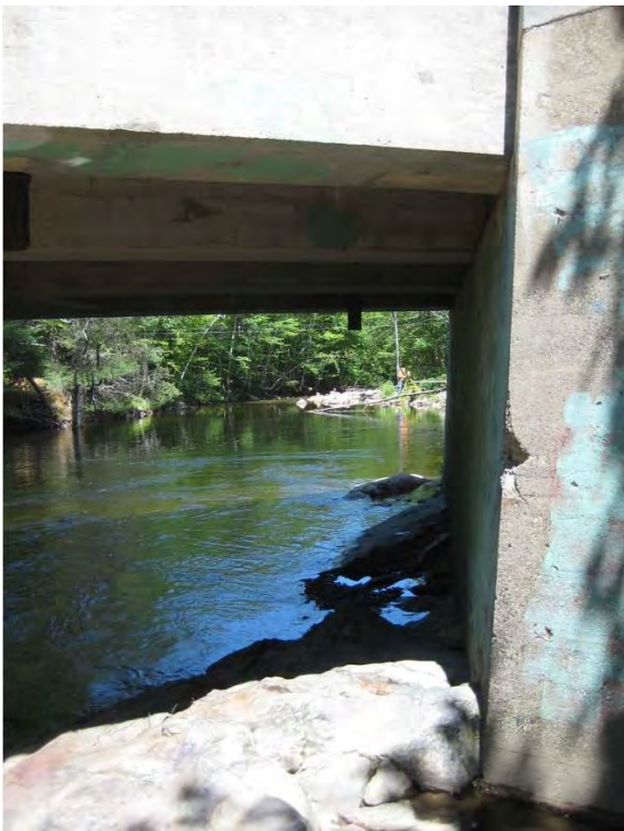
Figure 11. Looking downstream through bridge. Easterly or right abutment. Note scour hole downstream. Abutment founded on rock.
