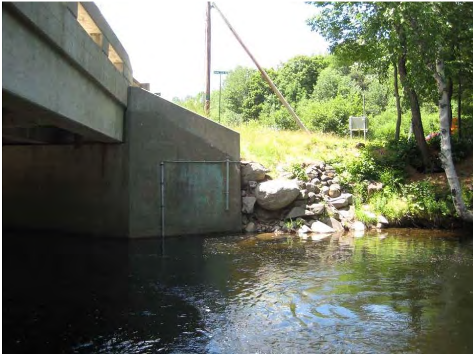
Figure 13. Downstream left/westerly abutment. Note abutment projects into flow.
