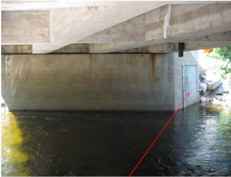
Figure 5. Left or westerly abutment with stream gage installation on downstream wing.
