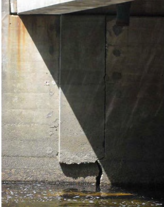
Figure 10. West abutment. Note cracking. Maine DOT inspection photos note cracking and rotation of abutment.
