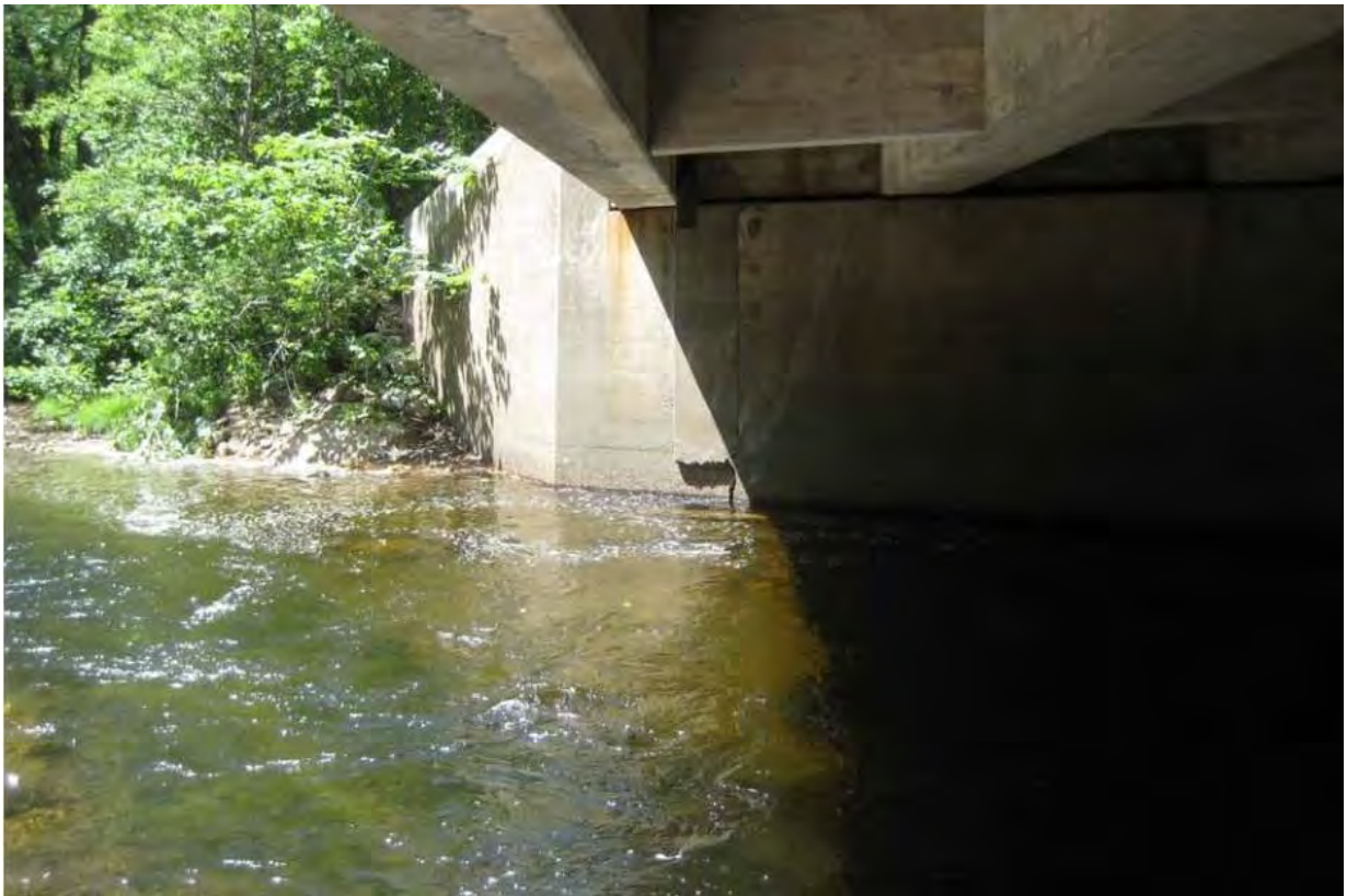
Figure 7. Looking at west upstream abutment. Note that abutment encroaches into main channel.
