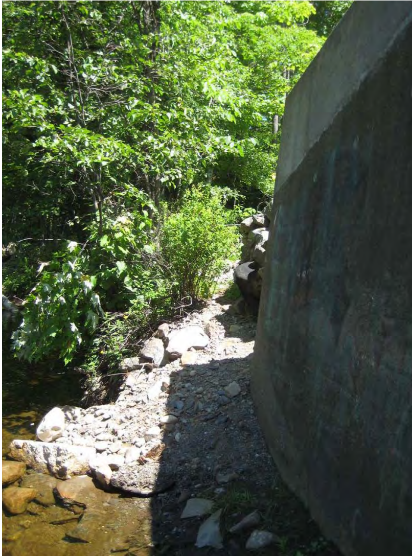
Figure 14. Upstream end of left/westerly abutment. Note projection into stream.
