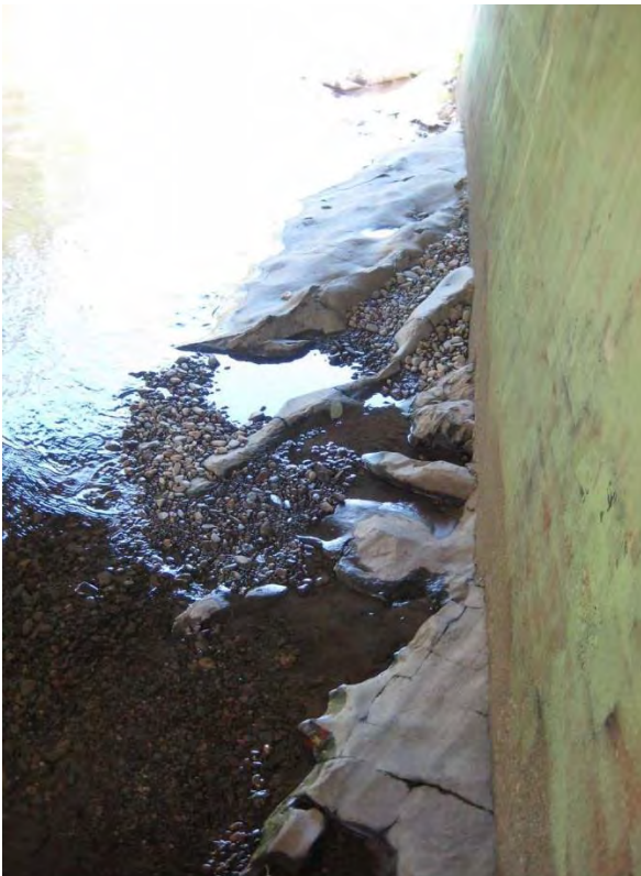
Figure 9. Right or eastern abutment set on rock.
