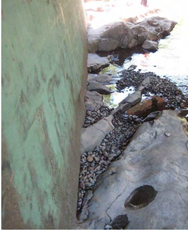
Figure 12. Right/East abutment looking upstream. Note abutment founded on rock.
